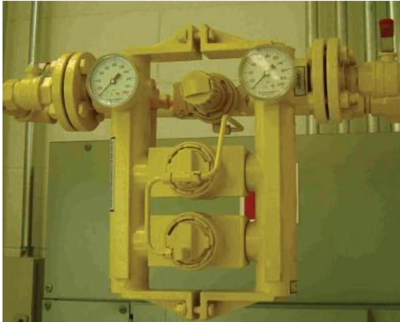
**Figure 25.** Pneumatic Flow Controller
